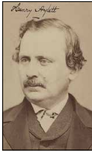
Figure 3: Patrick Henry Aylett, addressee and victim of the Capitol Collapse of 1870.
